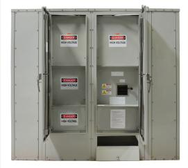
Solution for temporary remote connection of a facility's permanent generator to a load bank
